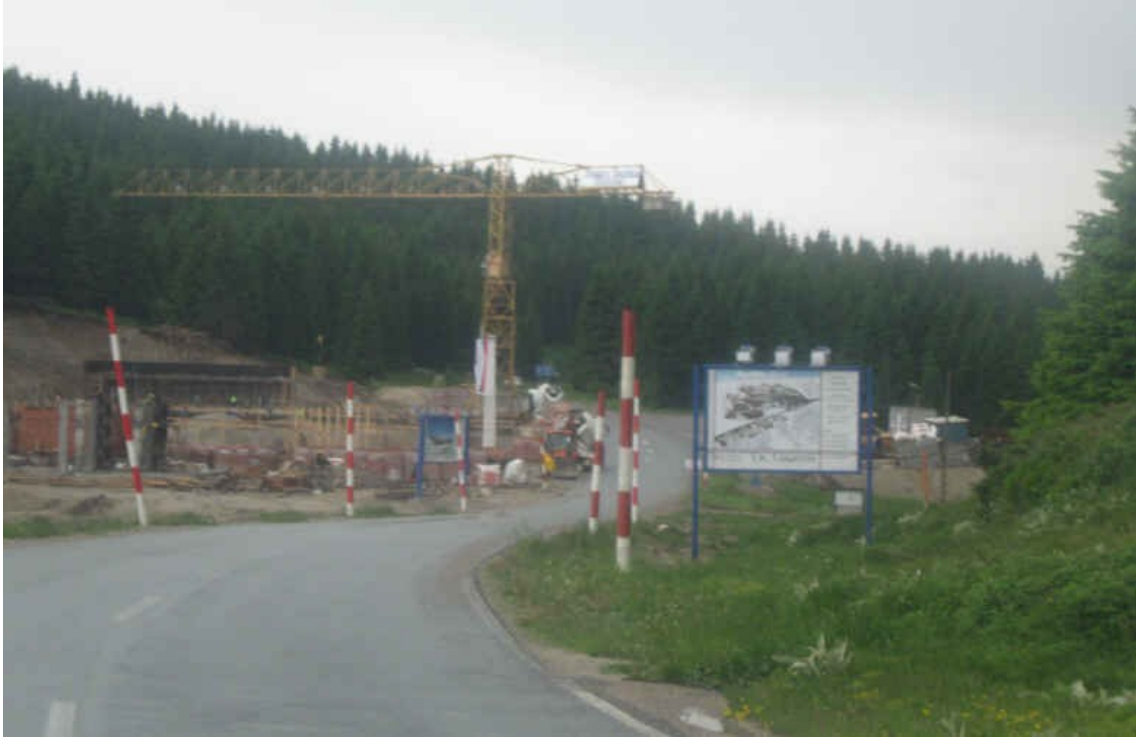
Resort under construction, in 2010
